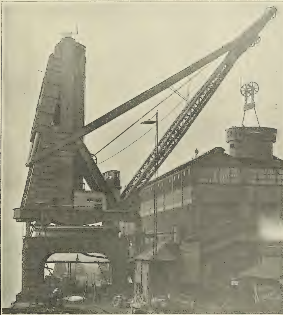
GENERAL VIEW OF THE NEW ELSWICK CRANE HANDLING A 12-INCH TURRET.
